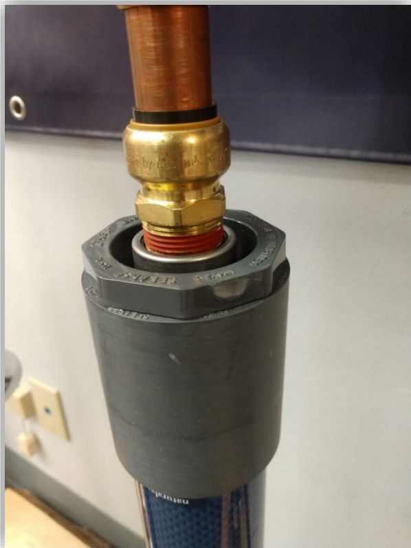
IN-LINE INSTALLATION (SharkBite™ Option Shown)
